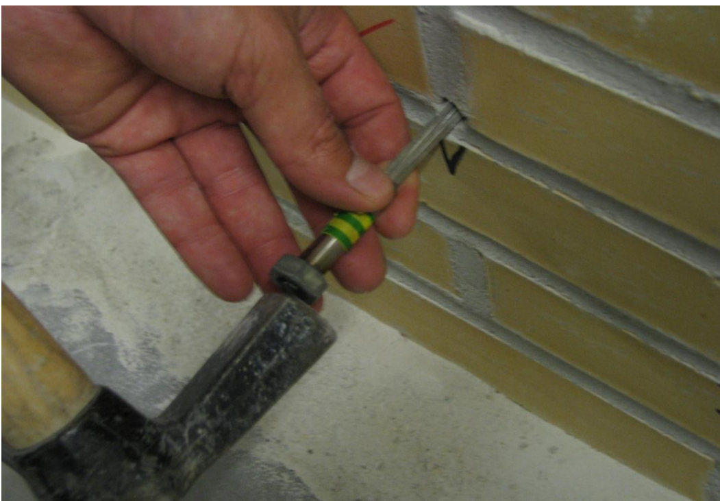
Figure 5. The X-drill is usually embedded 20-30mm in the joint.
