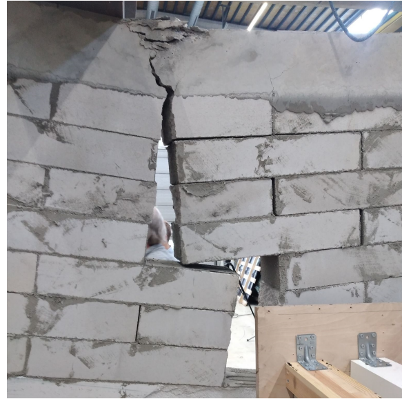
(b) Central crack from the back
