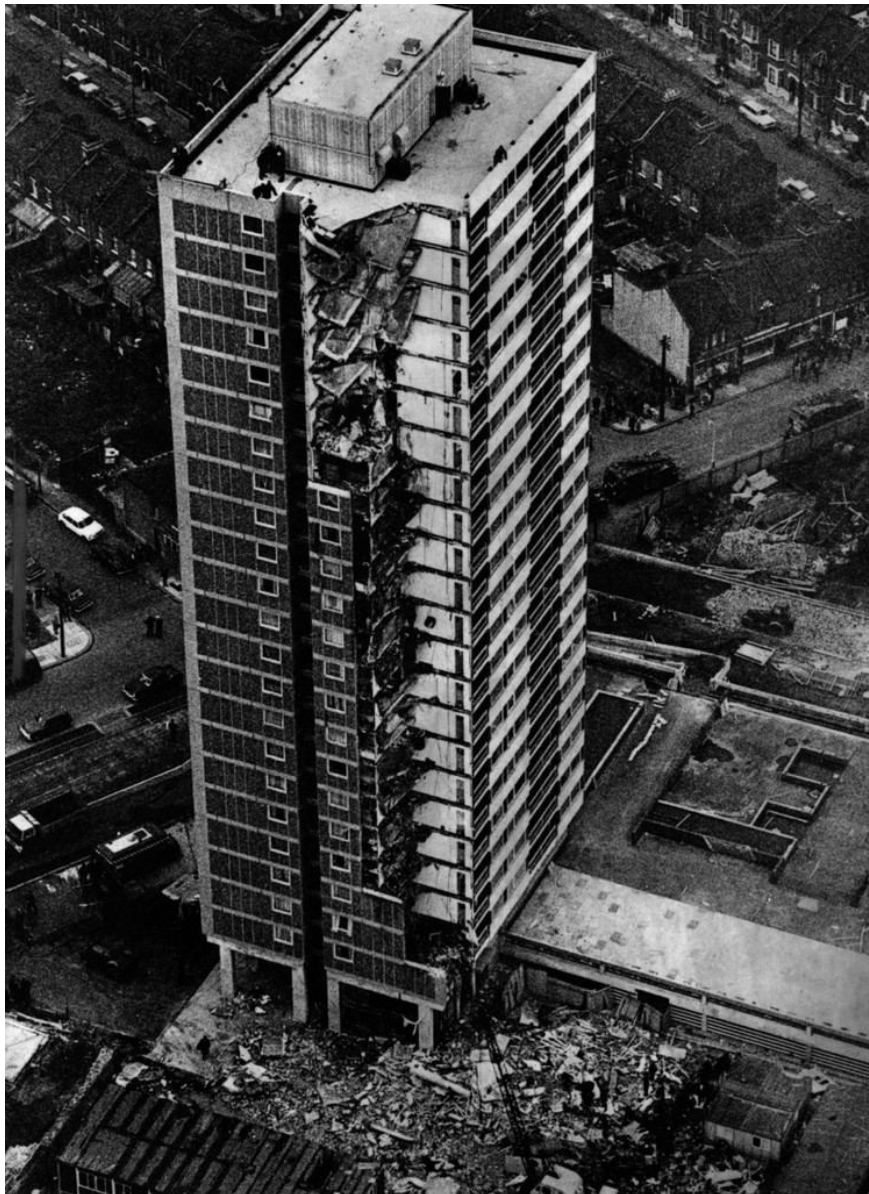
Figure 1: Progressive collapse at Ronan Point in 1968
