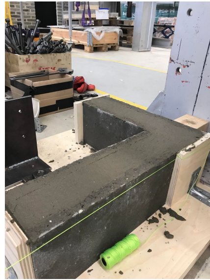
(b) Casting of concrete foundation
